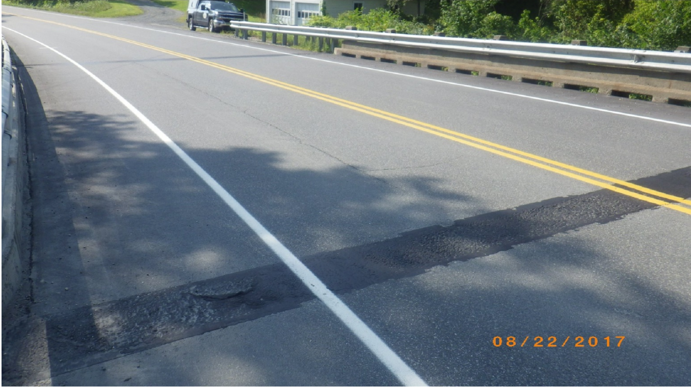
Looking south over the bridge.
