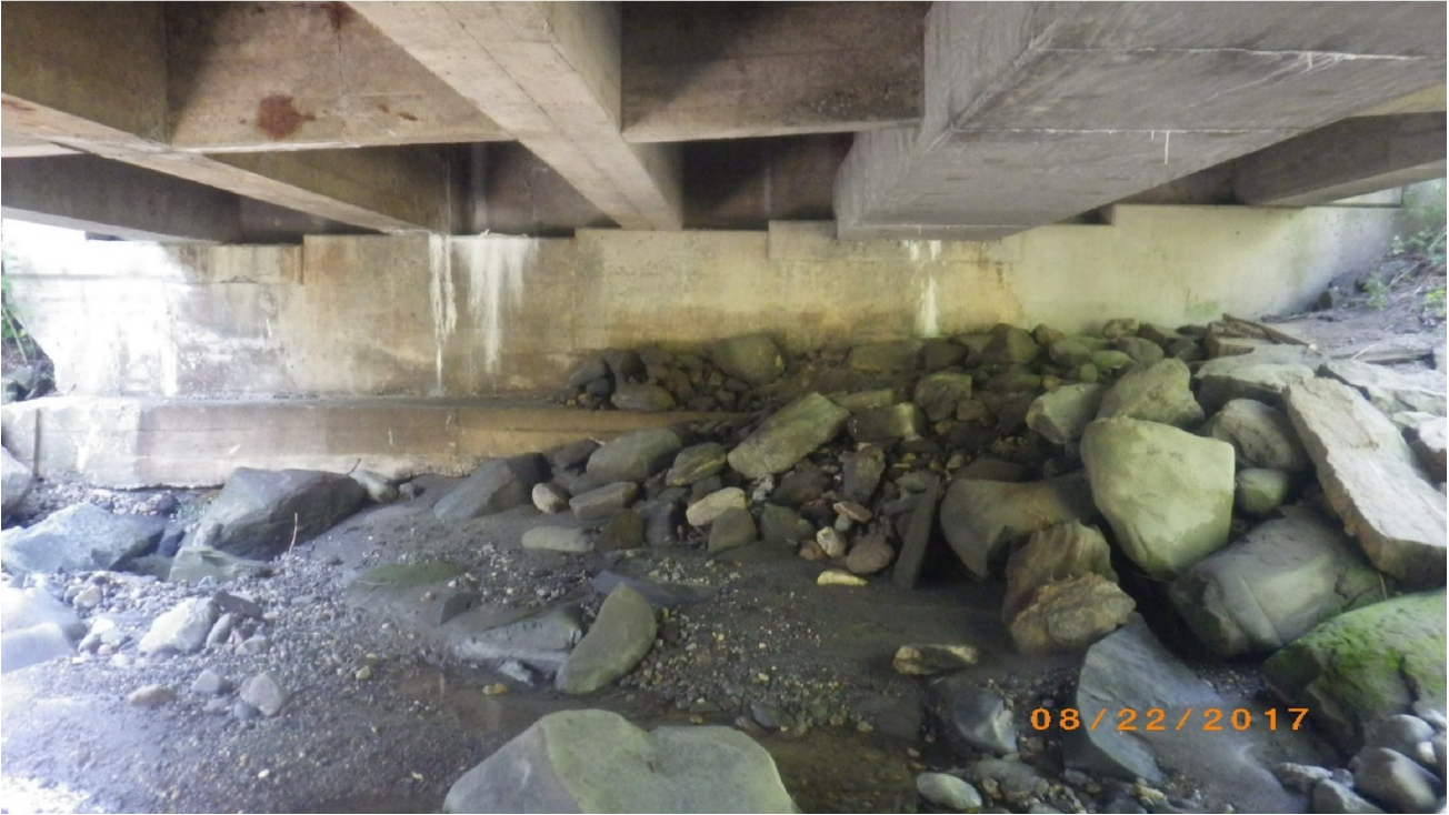
Southern abutment condition.
